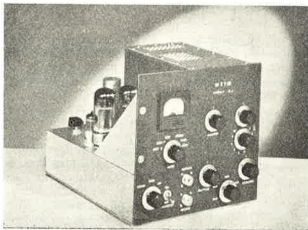
Fig. 1 — Front View of the 50-watt Mobile Transmitter.
